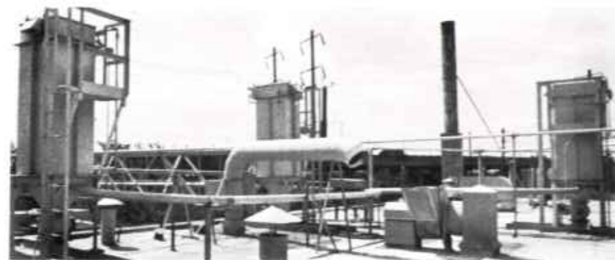
(left) Uni-Cage V/C Product Collector discharges into holding bin mounted below. Part of a TransVair Pneumatic System.
