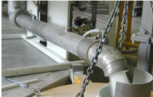
TiO 2 material discharging from a STINGER® conveyor into a dispersion mixer
